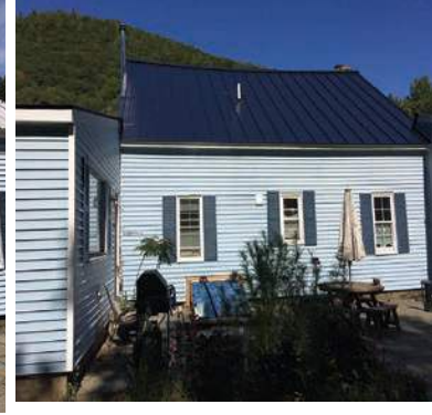
Roof repair, after
