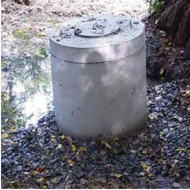
Well cap repair, after
