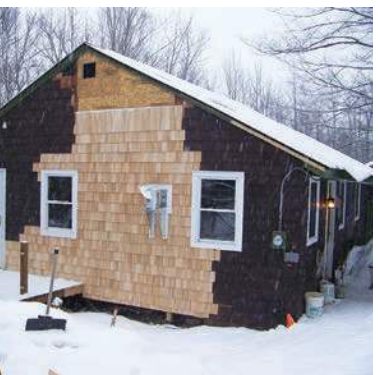
Siding repair, after
